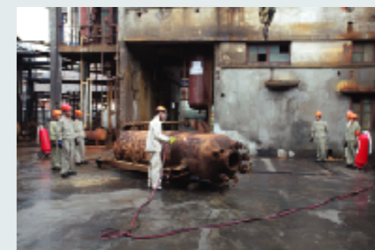
Dismantling of CFCs production equipment
