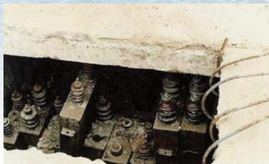
典型的含多氯联苯电力装置封存点（石棺封存） Typical sealing location (sealed in kistvaens) of PCBs-containing electric equipment
